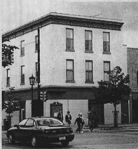
The historic storefront of this building has been filled in with masonry. Lack of storefront glazing discourages pedestrian involvement.
