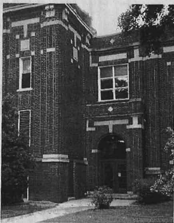
The original steel windows have been preserved in the doorway. The upper level windows are inappropriate replacements. The sash do not match the originals in profile or color. Opaque, colored glass should not be used.
