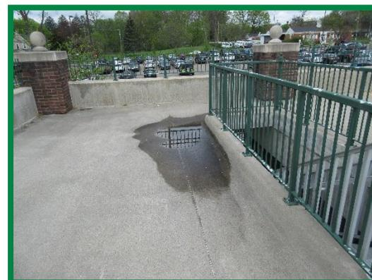
Water ponding was observed at the Upper Level Adjacent to the southwest stairs. This ponding could be relieved by minor re-profiling or installing a supplementary floor drain.
