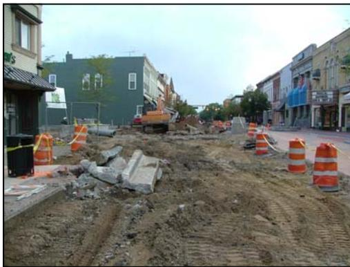
**Mary Alexander Court** – The concrete road base will be poured on Mary Alexander Court. Brick pavers will be installed on top of the concrete road base. Once the pavers are completed asphalt will be laid on the east and west ends of the bricked street. Mary Alexander Court will be closed to through traffic during this period
